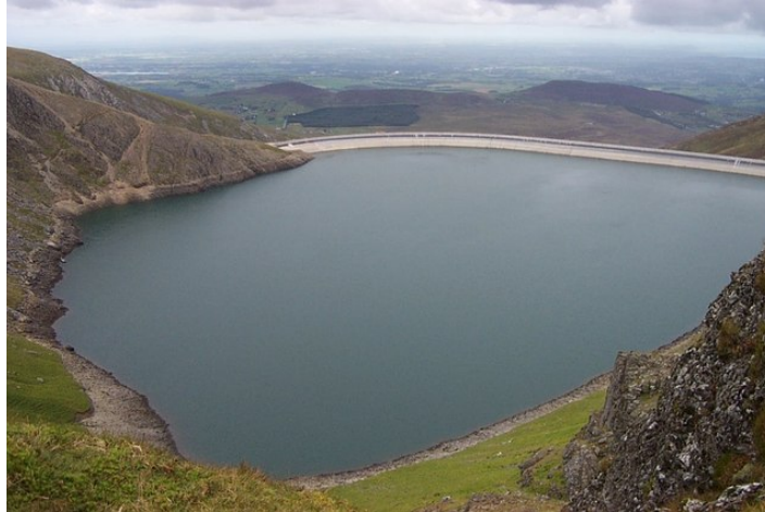
Figure 1 Top reservoir of Dinorwig, Wales PSP, 1.890 GW, 9.1 GWh. Source: © Copyright Terry Hughes, licensed under this Creative Commons Licence
